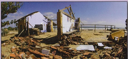
Damage to buildings from the tsunami.
