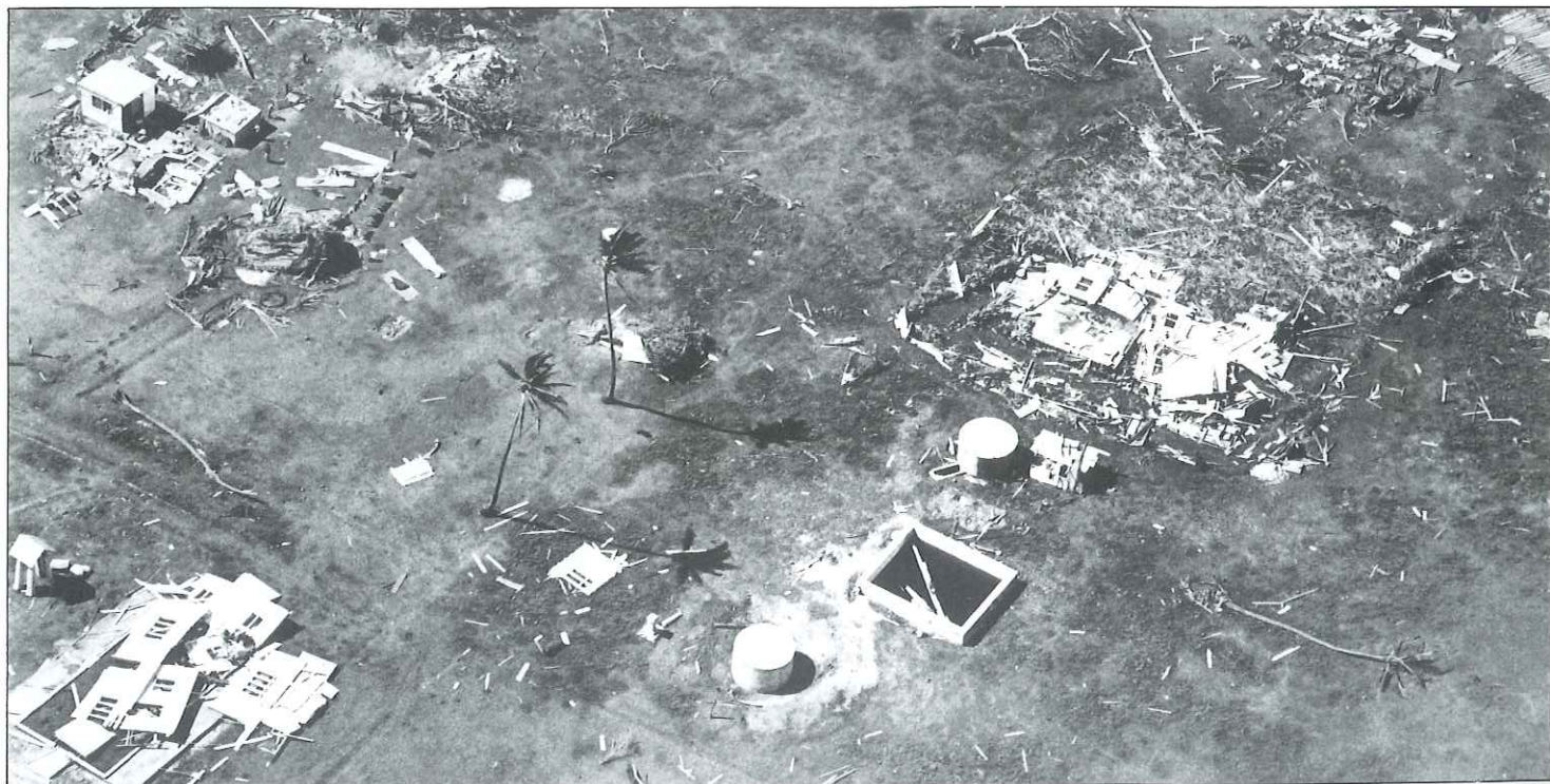
An aerial view of tropical cyclone damage in Tonga.
