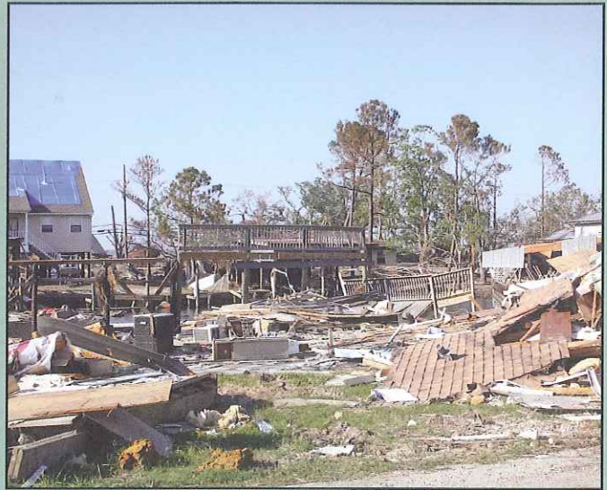
Heavily damaged homes.
